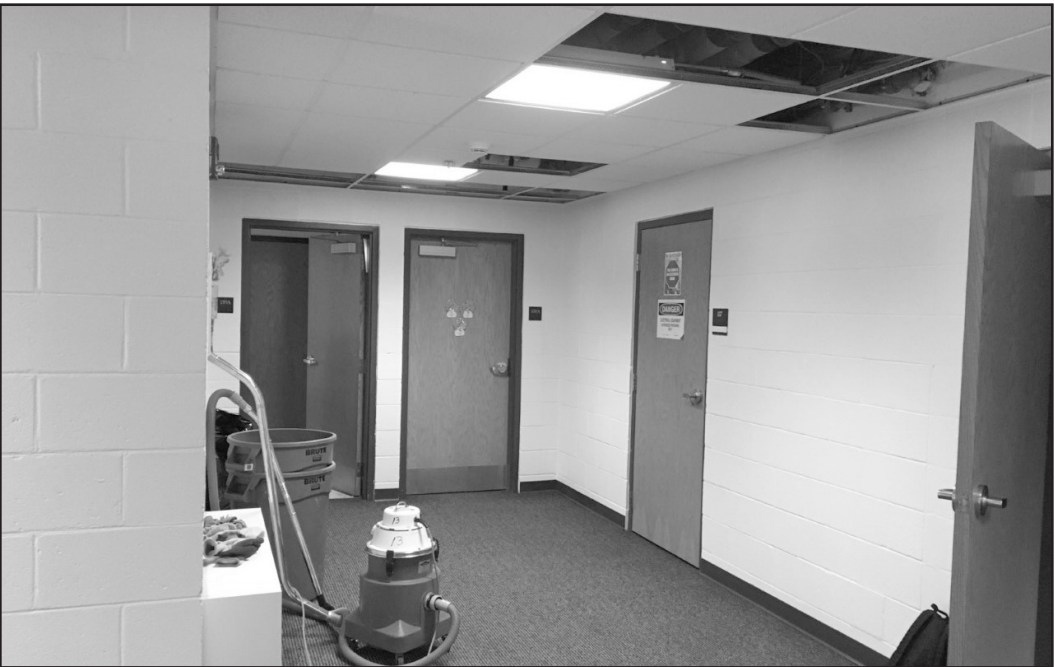
Water damage on the first floor below the room where the fire occurred.
