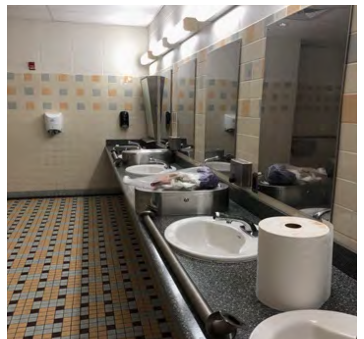
Work is currently being done in the boys bathroom due to the recent vandalism.
