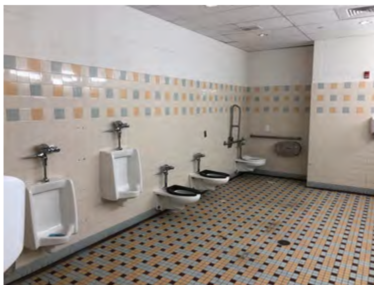
Vandalism has caused the closure of the boys bathroom in the math hallway. Stall doors, sinks, and toilets have all experienced tampering. The stall doors are currently removed as Amity works to repair the bathroom.
