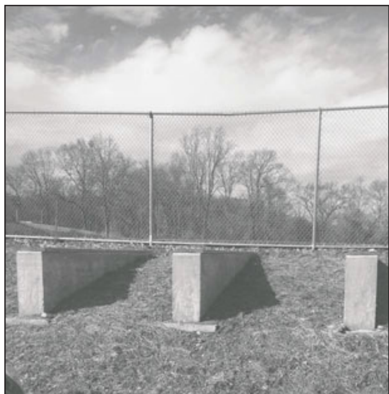
IMPROVEMENT Pictured are the foundations for the new bleachers Westhill will soon be receiving for their fans to sit on. Photo by Nicholas Zarrilli / Managing Editor.
