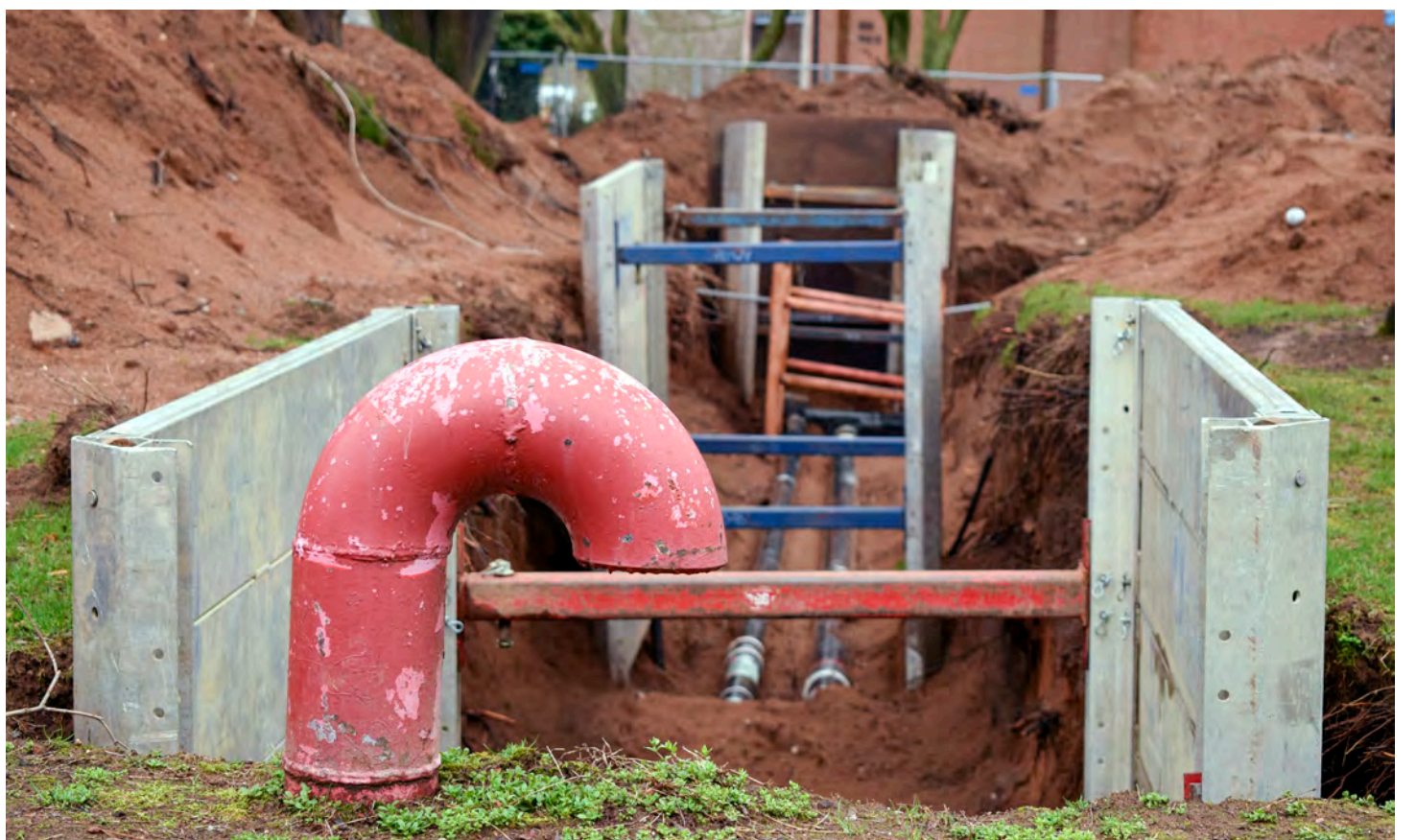
Piping placed between Earl Hall and the Lyman Center to repair and renovate the school's heating system.
