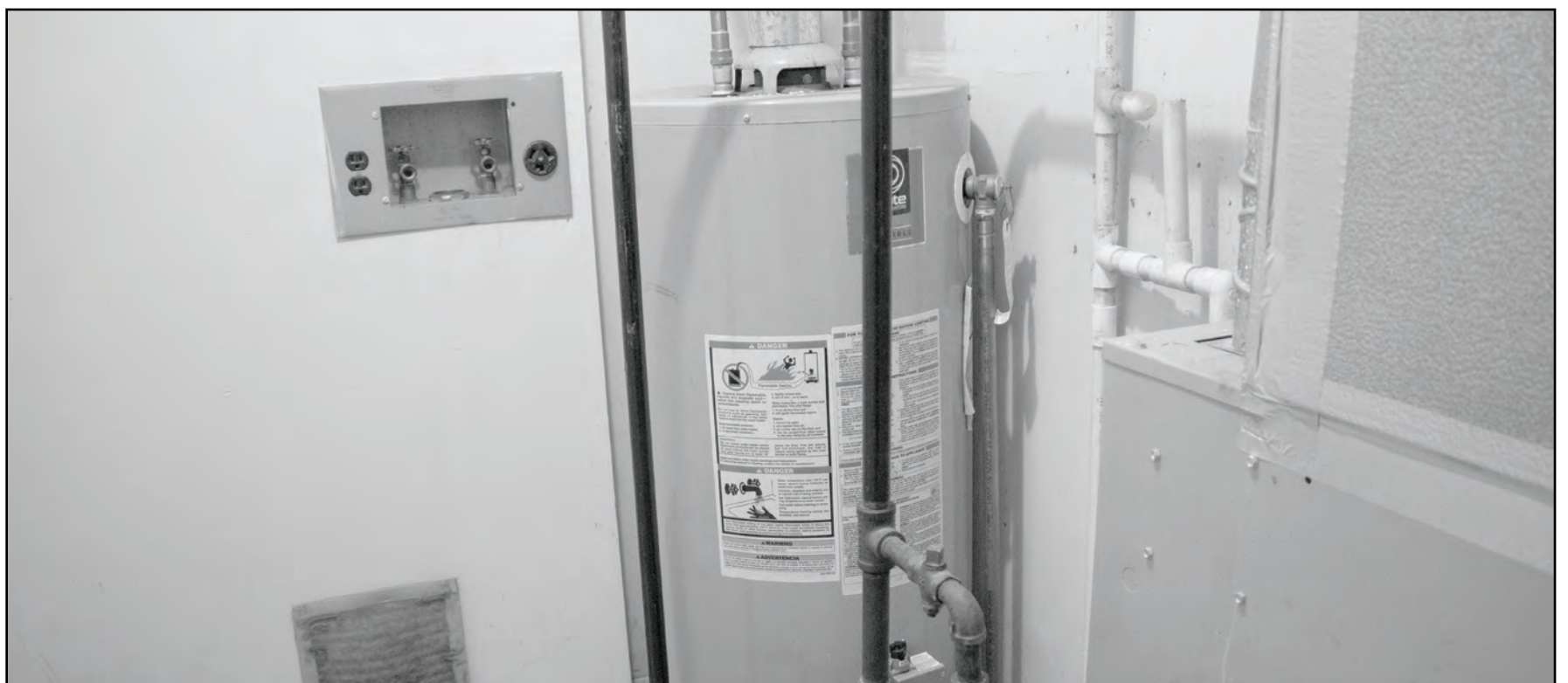
A water heater at one of the North Campus townhouses that need servicing at times to relight the flame that fuels the heating system.
