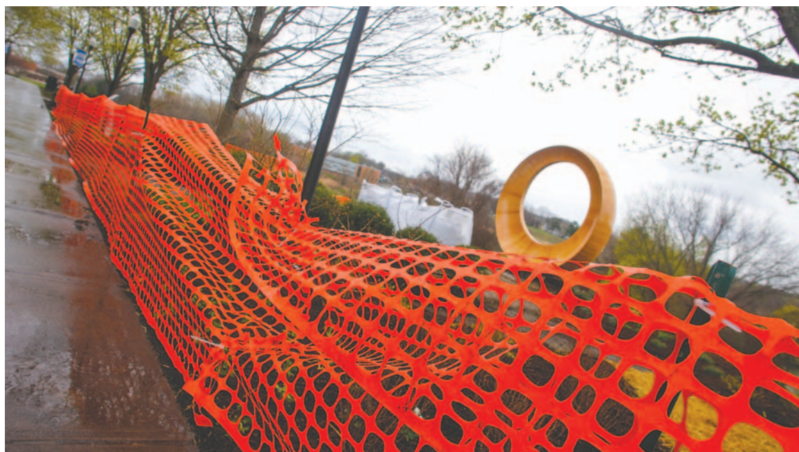
Temporary construction fence circling the perimeter of the garden.
