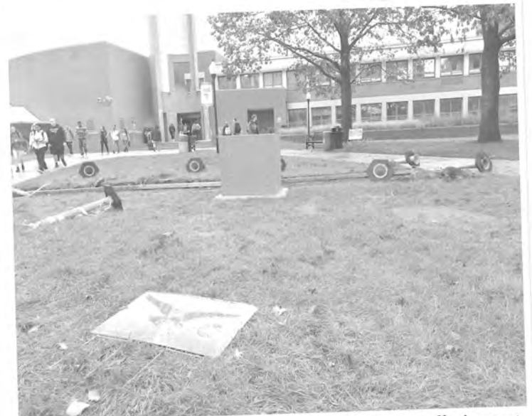
Nov. 6: No installation yet
