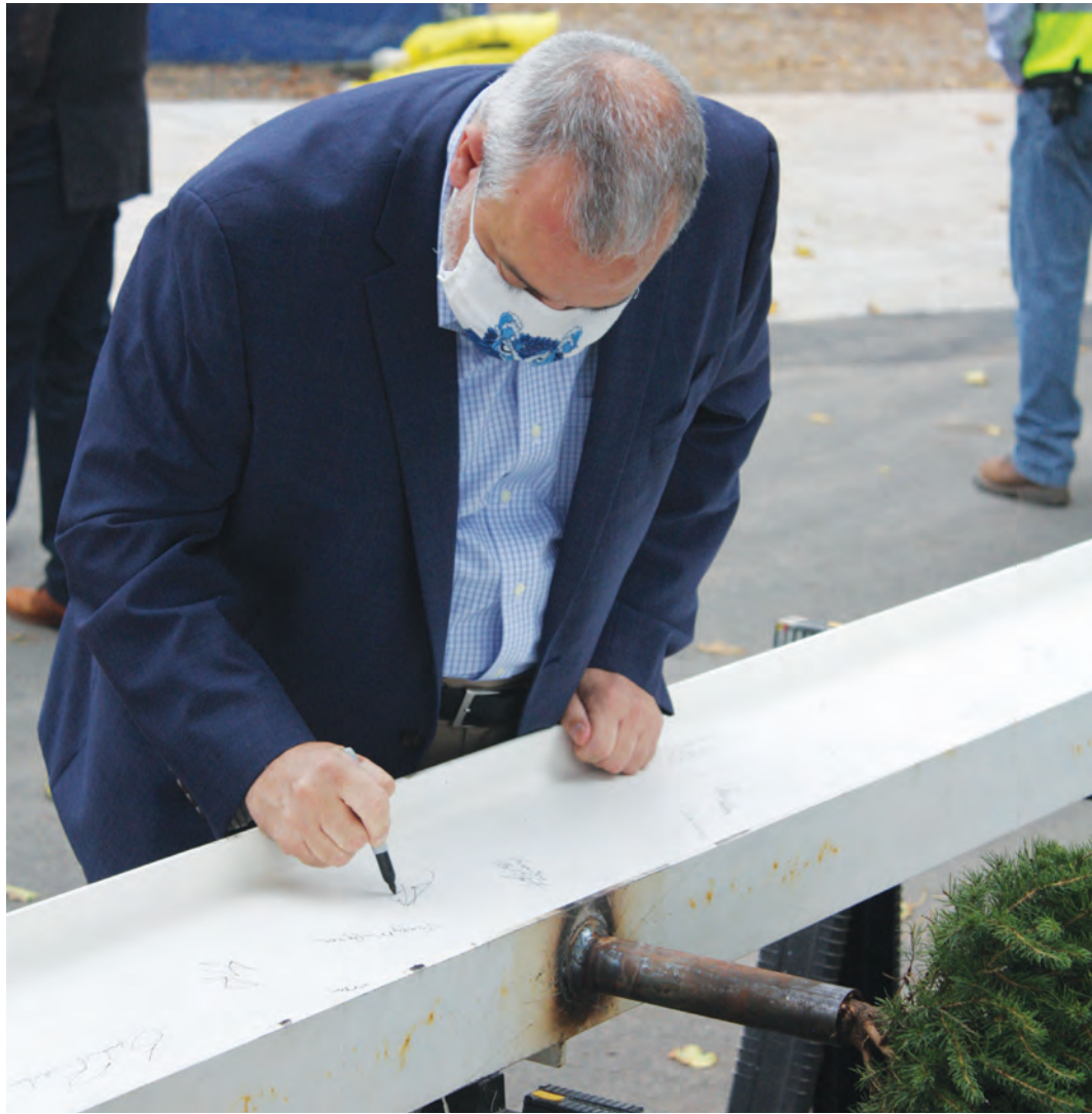
President Joe Bertolino signs his name on the final beam before it is placed on the steel structure.
