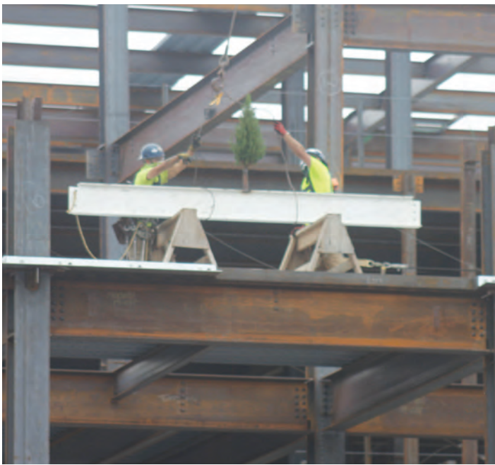
The final beam is received by construction workers on top of the steel structure.
