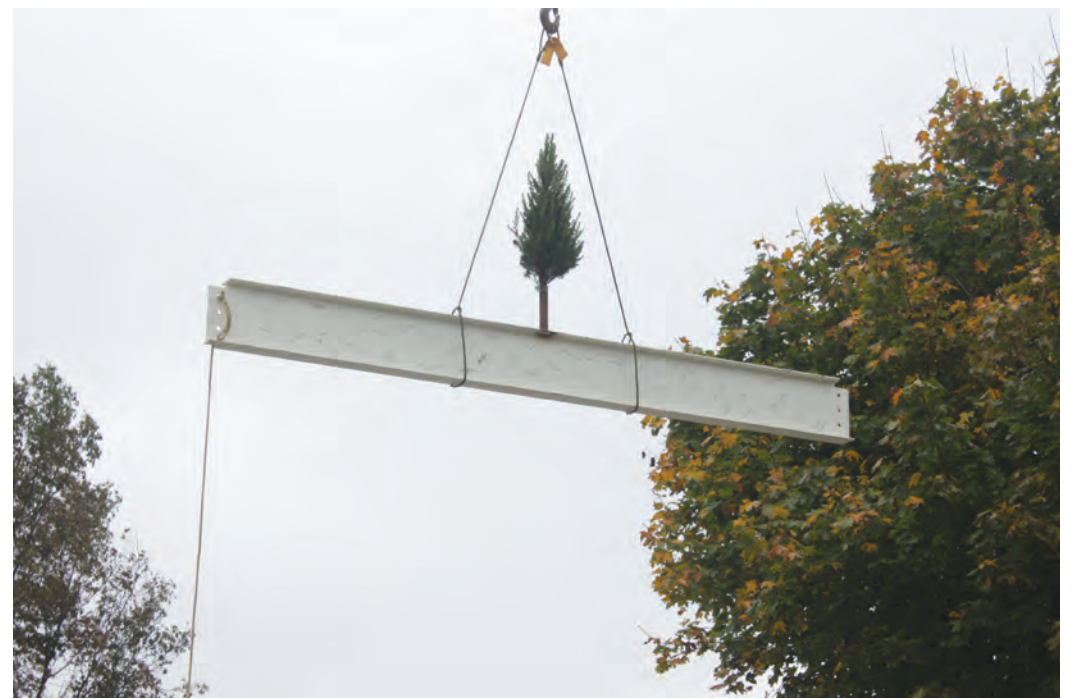
The final beam, topped by a tree, is lifted by a crane to be placed on top of the future Health and Human Services building.
