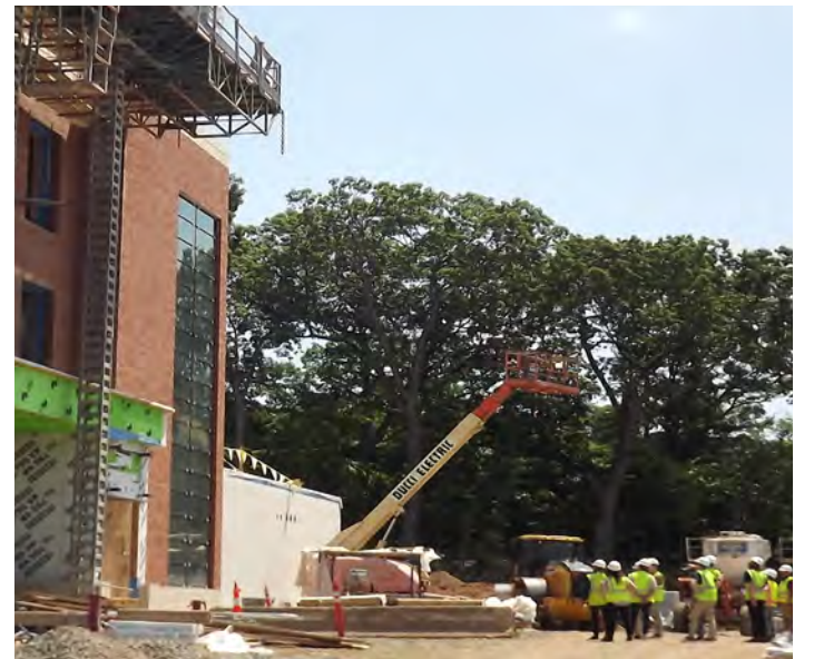
Construction works gather around the side of the Barack H. Obama Magnet University School.
