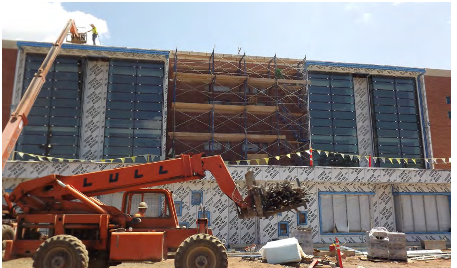
A construction worker operated a lift while another worked on the roof of the Barack H. Obama Magnet University School.
