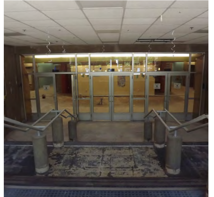
The entryway to Connecticut Hall while undergoing renovations over the summer.
