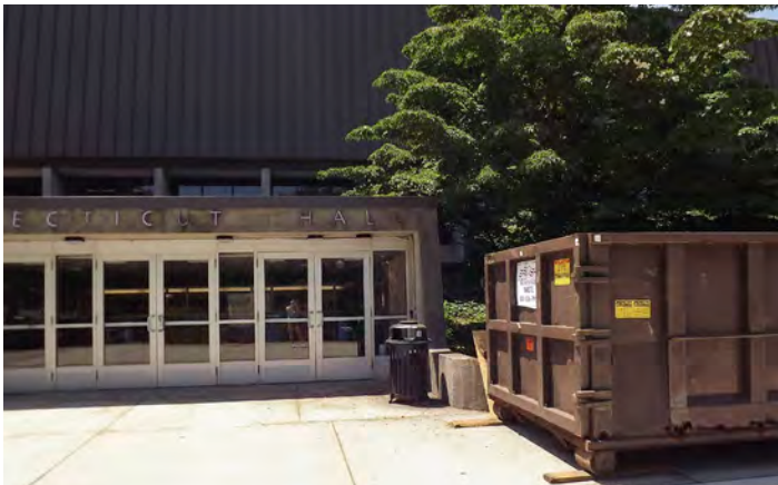
A dumpster in front of Connecticut Hall during renovations.
