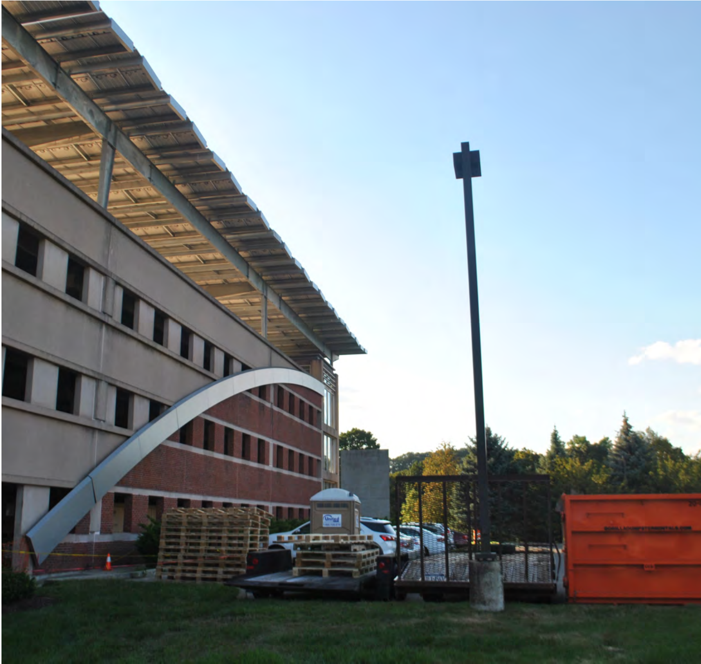
Solar panels and construction supplies at the rear end of the Fitch Street Garage near Davis Hall.
